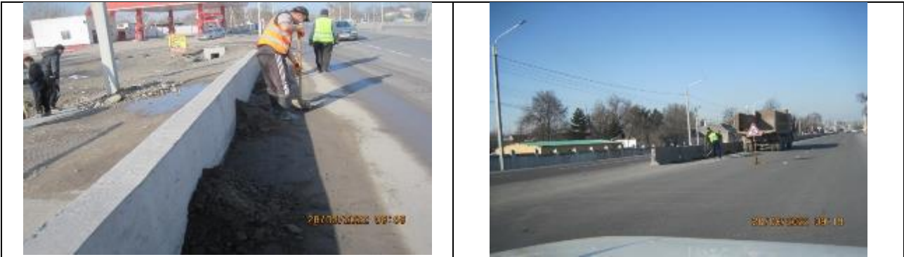
Figure 28 Cleaning of area near parapets from earth waste and removal of waste from the road
