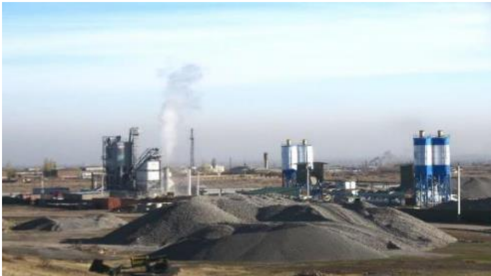
Figure 18 Production site. Concrete mixing plant. Asphalt Bitumen Plant
