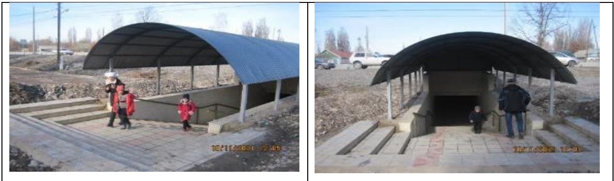
Figure 10 Underpass in the Novonikolaevka
