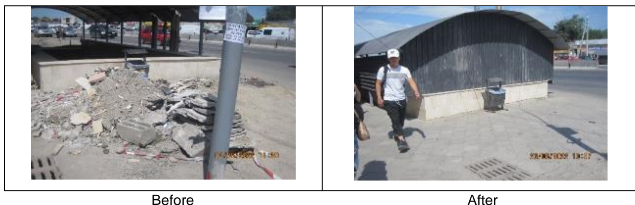
Figure 57. Construction waste near the underpass under construction in the center of the Sokuluk.
