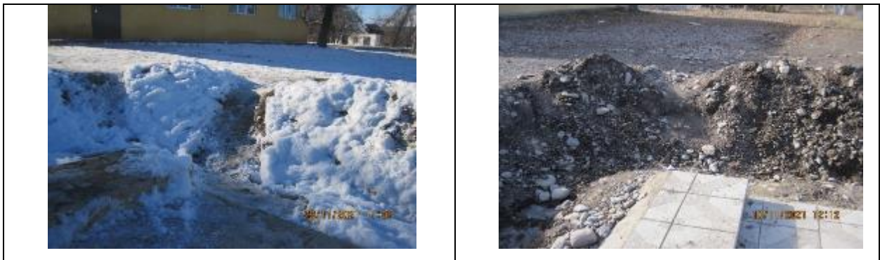
Figure 32 Construction waste around the underpass located near the school in the village of Novonikolaevka.
