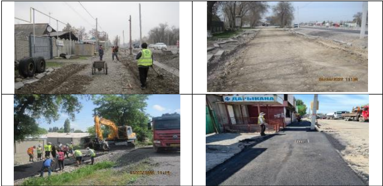
Figure 6 Construction of sidewalks
