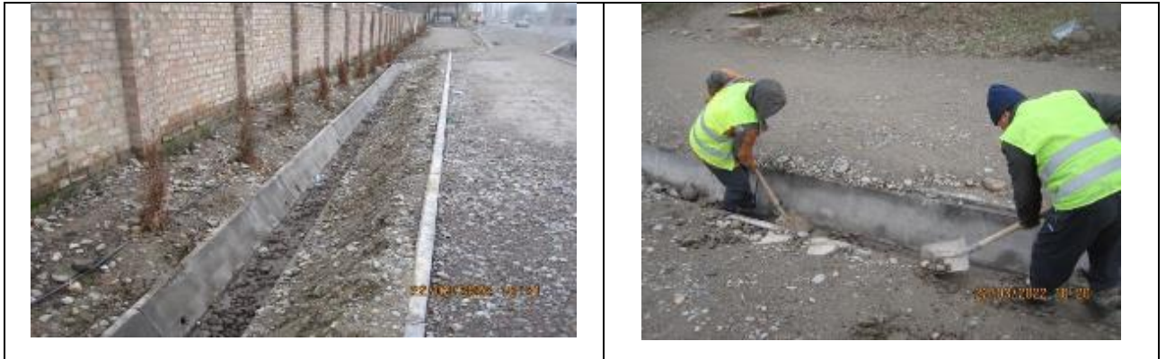
Figure 29 Cleaning of side culvert ditches
