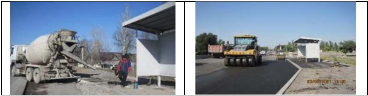
Figure 3 Asphalting of bus bay areas.
