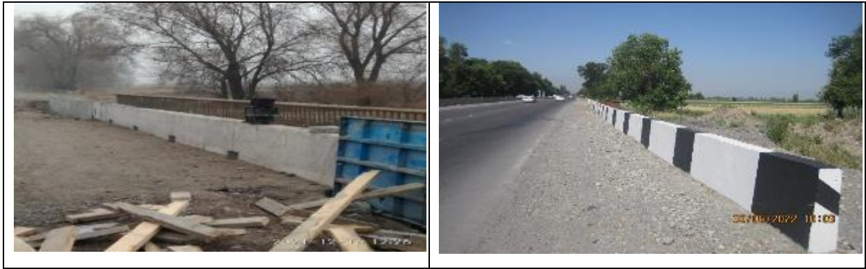
Figure 11 Construction of a wheel-safety parapet barriers at the Jelamysh river
