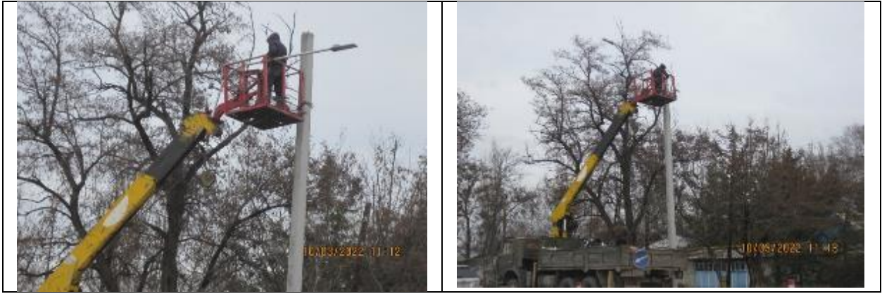
Figure 8 Street lighting works. Installation of lamps
