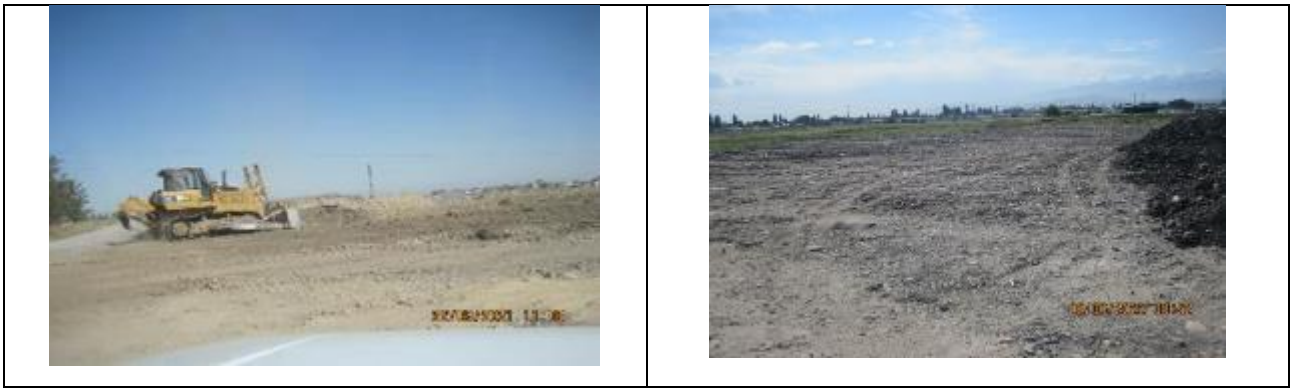
Figure 54 Storage and levelling of unsuitable soil for further use in the village of Voенно-Antonovka.
