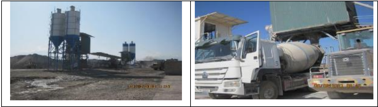
Figure 22 Filling the concrete mixing machine with concrete
