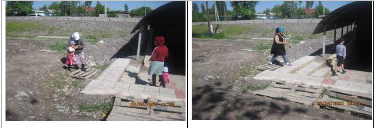
Figure 33 Violations near the underpass located opposite the school in the village of Novonikolaevka
