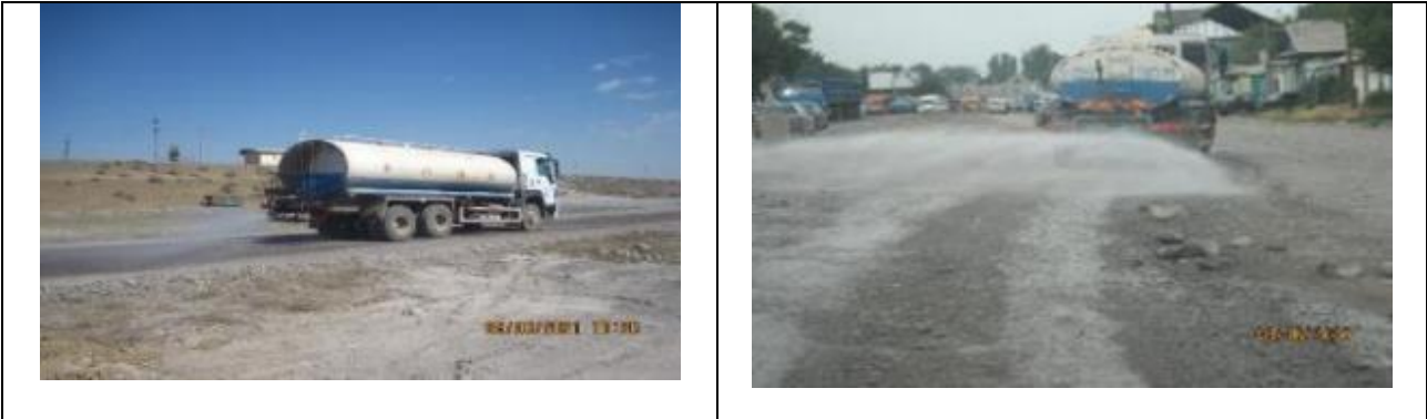
Figure 27 Water sprinkling works. Road to the production site and at the road construction site in the Voенno-Antonovka
