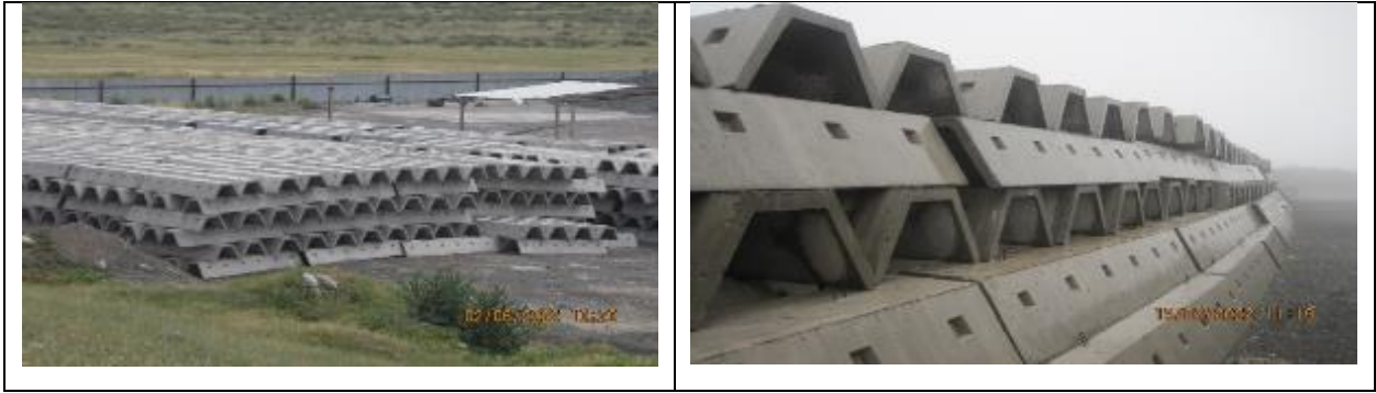
Figure 19 Prepared reinforced concrete structures
