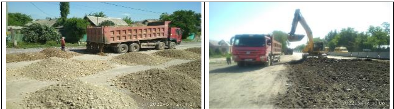
Figure 12 Levelling of roadbed in the village of Voенno-Antonovka
