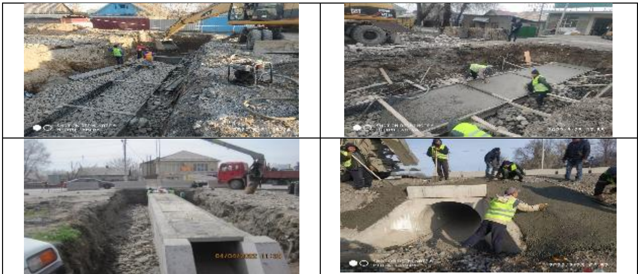
Figure 14 Construction of culvert pipes
