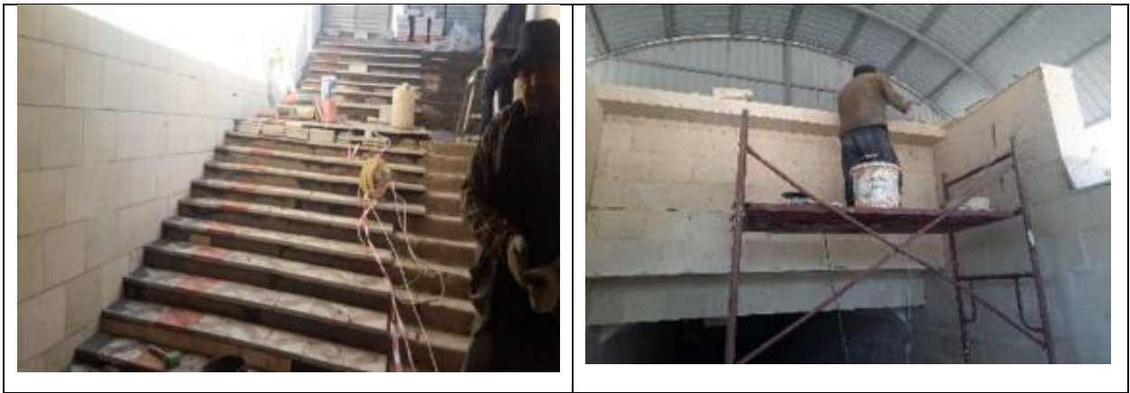
Figure 9 Completion of construction works in underpasses
