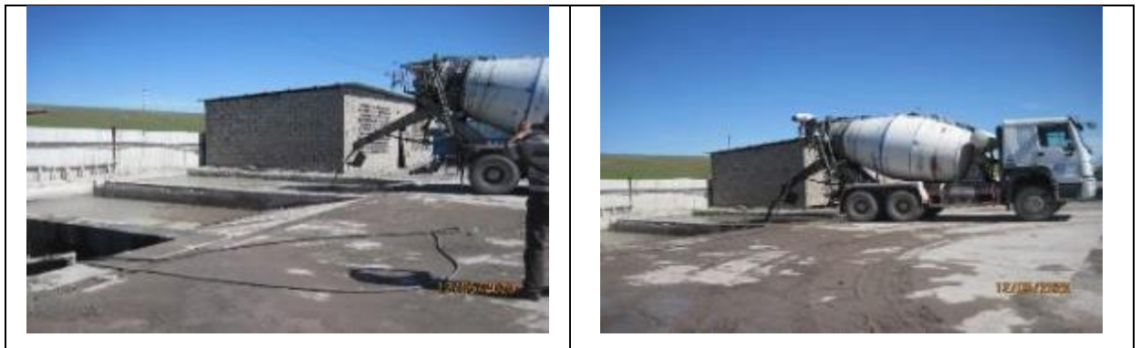
Figure 42 Washing of concrete mixer trucks.
