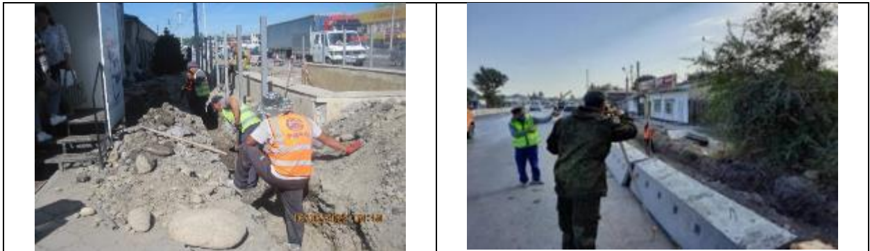
Figure 4 Installation of side culvert ditches
