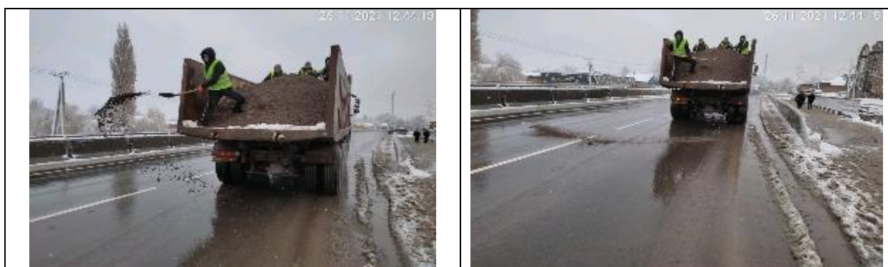
Figure 26 Spreading sand on the road. Ice control.
