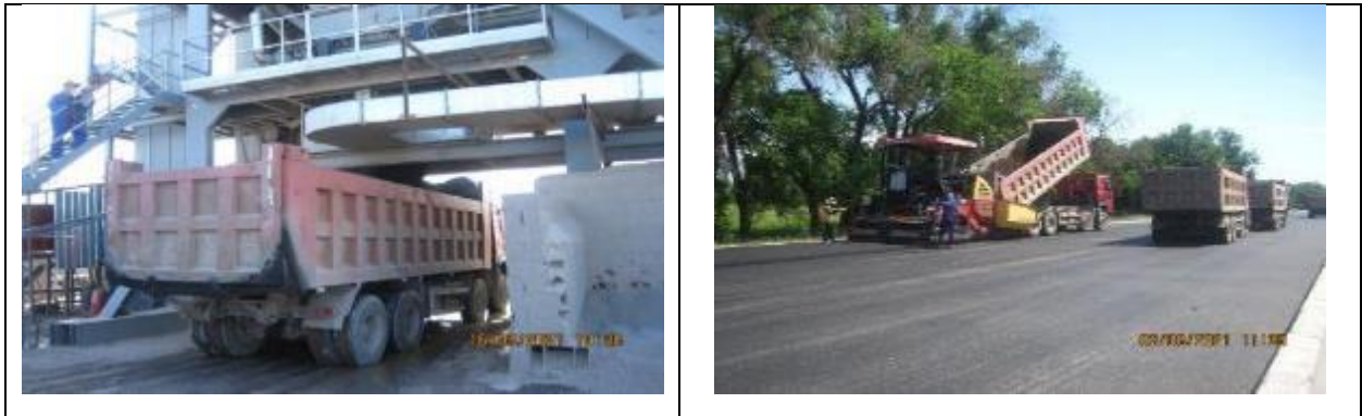
Figure 23 Loading of asphalt mixture into dump trucks and unloading into asphalt pavers.
