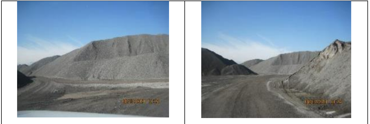
Figure 39 Prepared gravel material for concrete and asphalt production
